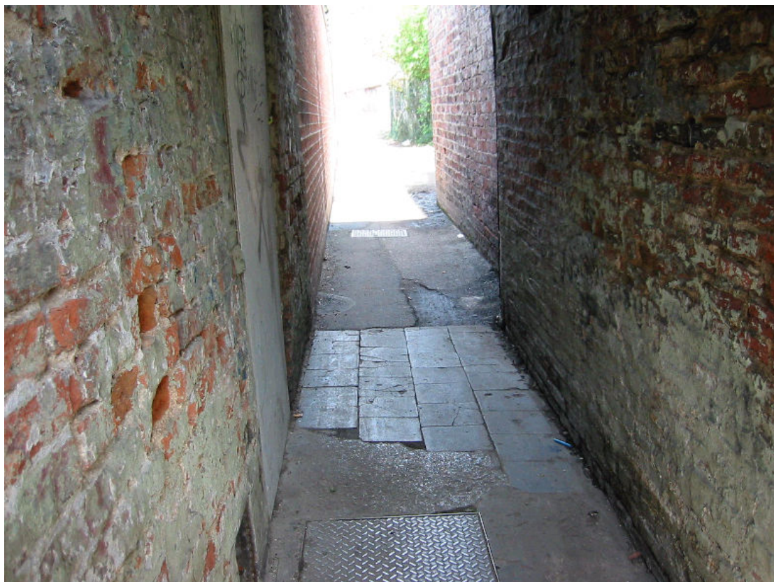
Figure 2: Beneath buildings off Clifton, note existence of Utilities
