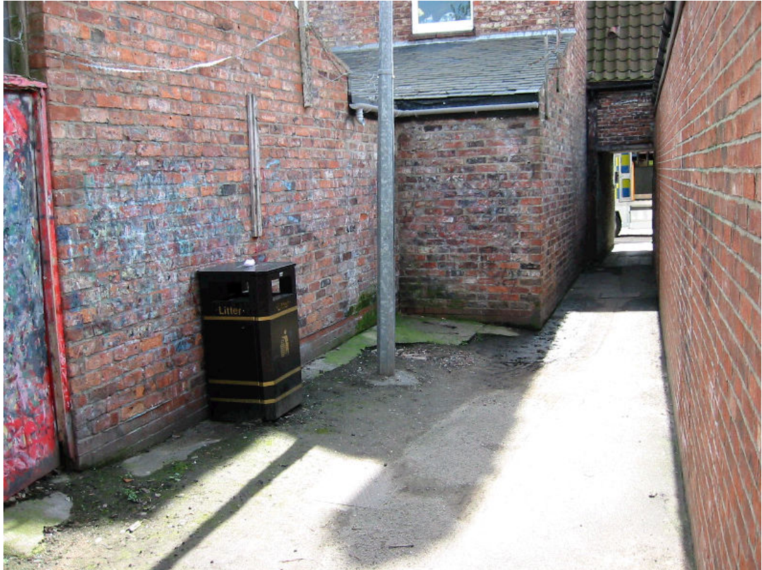
Figure 3: Lighting Column and Council litter bin
